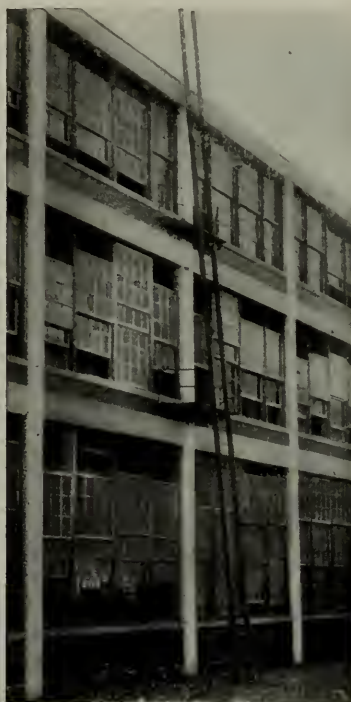
Permanent Fire Ladder Installation
