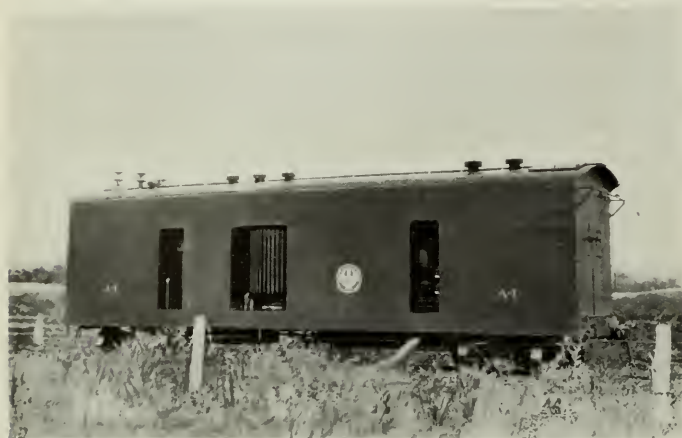
Fig. 8. Portable Automatic Substation
