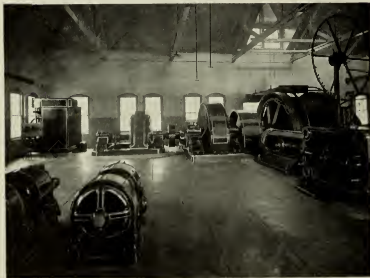
Fig. 2. Electric Hoist, showing Flexible Coupling and Drag Link. Liquid rheostat, tank and contactor control panel for hoisting motor are shown in corner of room
