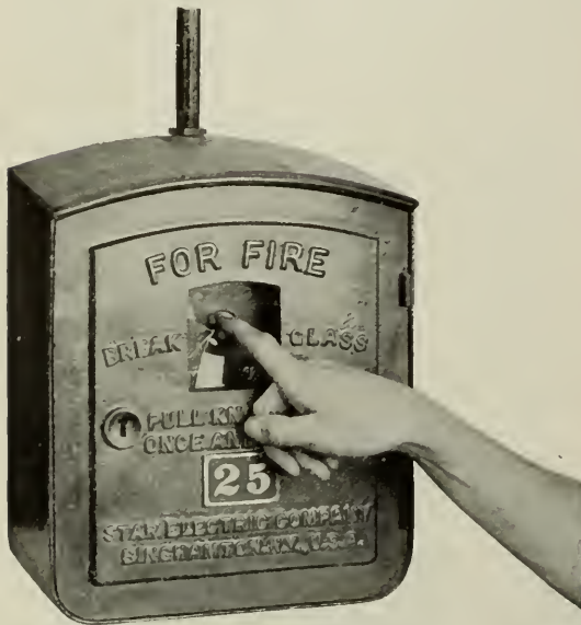
Giving Fire Alarm from Master Box
