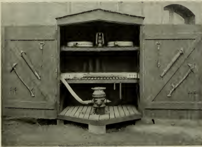
Interior of Hose House, Showing Four-way Hydrant, Hose, and Other Equipment
