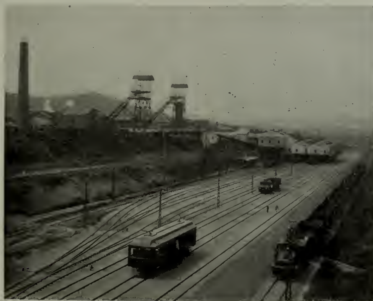
Fig. 3. Oyama Shaft and Screening Plant
