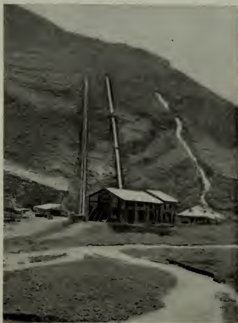
Fig. 3. Power House, Bella Vista, Peru. Elevation 12,500 ft.
