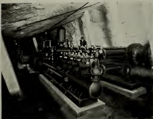
Fig. 7. Pump End of 1500-gallon Prescott Duplex Double-Acting Station Pump, Muscada Slope No. 4
