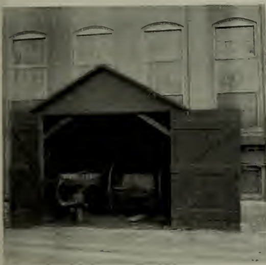
Hose House Containing Reel Cart
