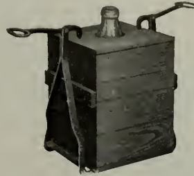
Devices for handling acid carboys. The destructive action of acid may lead to the case becoming rotten, so tongs are provided which reach under the box and would prevent the bottle falling even if the bottom came away entirely. When small quantities are required, the carboy is held in an inclinor which is easily tipped without danger
