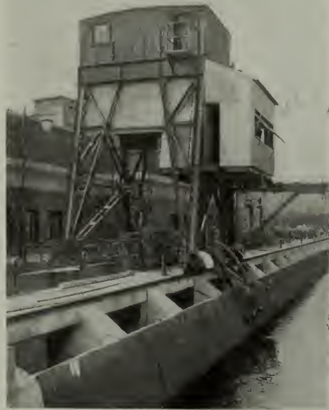
Fig. 5. Gantry Crane and Special Rack Raking Device
