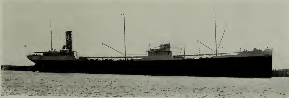
Steamship "La Brea" Powered with 2600-h.p. Curtis Turbine Driving through Alquist Reduction Gears
