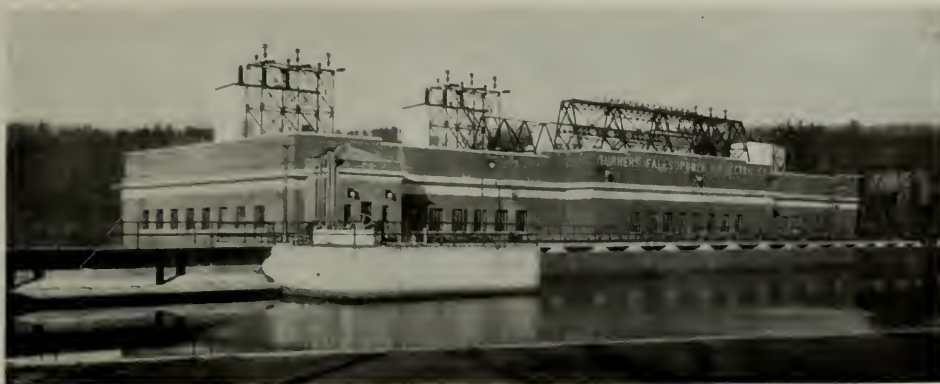
Fig. 2. View of Station from Canal Side
