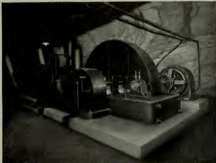
Fig. 6. Crank end of 1500-gallon Duplex Double-acting Prescott Station Pump showing enclosed Herring Bone Gear, Flexible Coupling and 300-h.p. Wound Rotor Induction Motor. Fossil Slope No. 8
