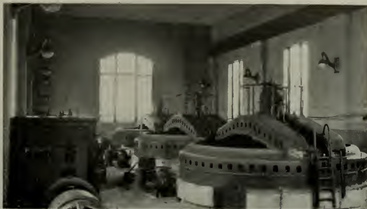
Fig. 8. General View of the Interior of the Automatic Generating Station. A Motor-driven Exciter is shown in the Lower Left-hand Corner
