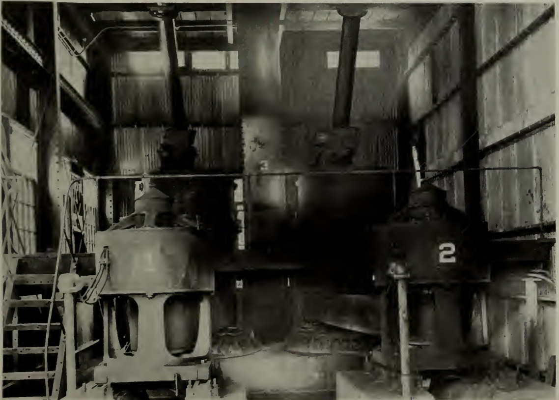
Fuller-Lehigh 42-in. Pulverizer Mills at Parsons Plant
