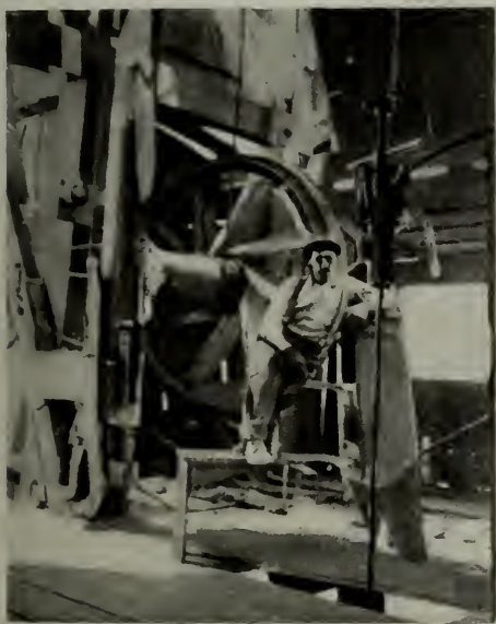
Fig. 5. Drilling a 1900-ft. oil well by electric power with standard cable tools in the Midway field in California
