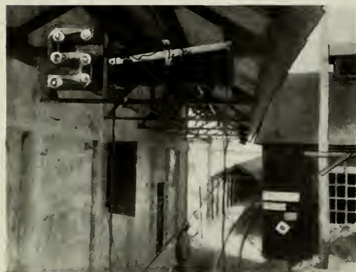
Fig. 23. Manually Operated Switch at Portal of Main Tunnel for Controlling Block Signal System
