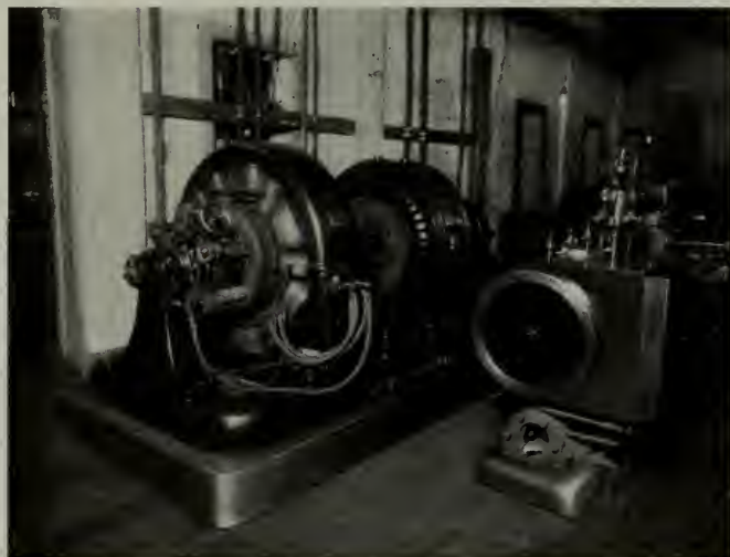
Fig. 14. Motor-generator Set Furnishing 500-volt Direct-current for Mine Locomotives
