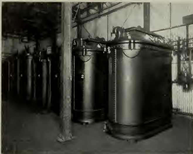
Fig. 4. View in Substation of Bunker Hill & Sullivan Company Showing Seven 650 kv-a. 60,000/2300-volt Transformers
