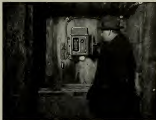
Fig. 26. Installation of Telephone
