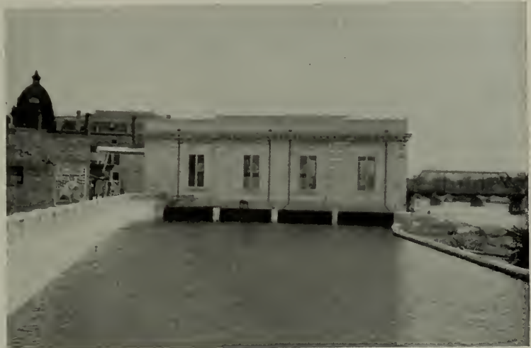
Fig. 2. Forebay Side of the Automatic Generating Station
