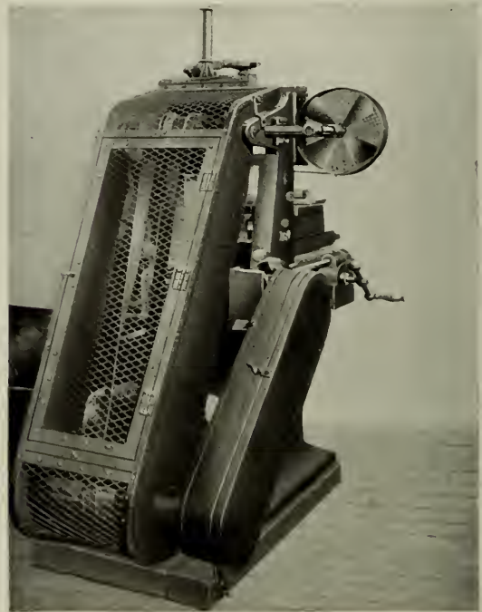
Belt Guard on Profiler
