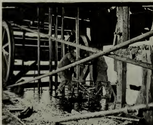
Fig. 8. Pulling tubing with motor drive in the Midway field in California
