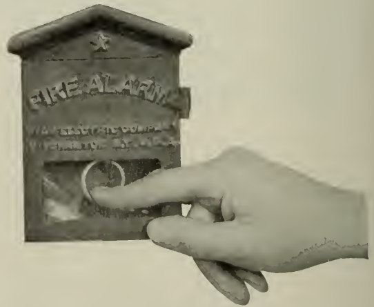
Giving Alarm from Auxiliary Box
