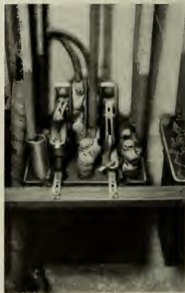
Fig. 10. Contacts for Alarm Bell Mounted on Back of Oil Switch. When Oil Switch is Tripped by Tell-tale Device at the Motor Pulley the Switch is Tripped and the Alarm is Sounded
