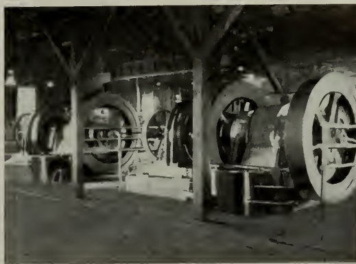
Fig. 9. The power station of the Crowley Oil and Mineral Co., Evangeline, La., showing two 75-kv-a. oil engine-driven generating units, now supplemented by a third
