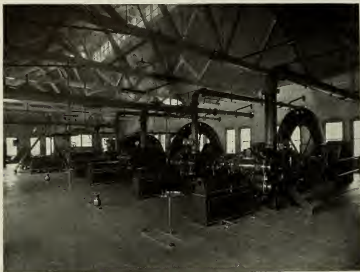
Fig. 4. Two Synchronous Motor-driven, Twin, Two-stage Air Compressors with Former Steam Ends Removed
