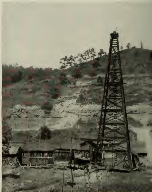
Fig. 1. Well No. 1, Henry Talkington lease, South Penn Oil Co., Folsom, W. Va. One of the first electrically operated oil wells in America
