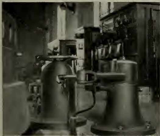
Fig. 7. Waterwheel Gate Control in the Foreground and Automatic Control Cabinet Panels in the Background
