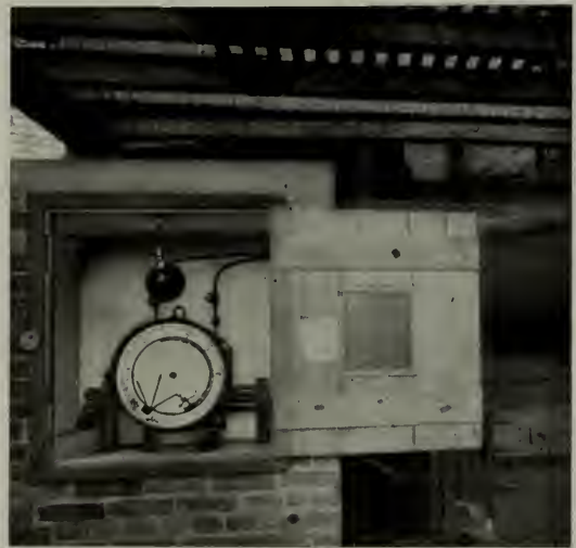
Fig. 4. Indicating Recording Integrating Flowmeter installed in a 14-inch line supplying steam to the mills of the Pennsylvania Steel Company, Steelton, Pa.
