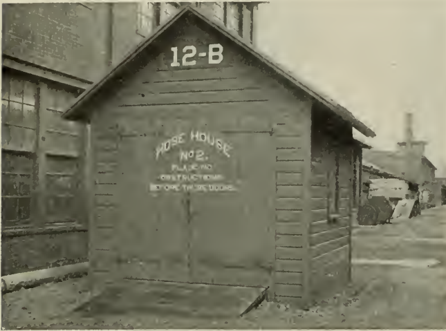
Typical Hose House
