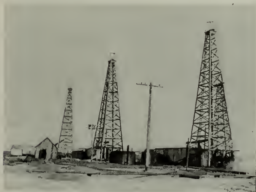
Fig. 6. A group of motor-operated oil wells in the Spindletop field in Texas. The farthest well is pumped by a jack operated from the middle well
