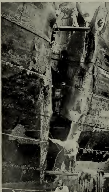
Fig. 1. Hole in Side of Steamship Caused by Collision. Arc Welding Set Used in Making Repairs
