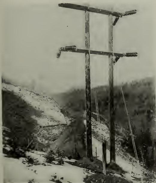
Fig. 3. 100,000-Volt Transmission Tower for Long Span
