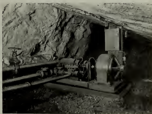
Fig. 8. 400-gallon 4-stage Centrifugal Pump, Driven by 100-h.p. Squirrel-cage Induction Motor for Furnishing Domestic Water Supply. Muscada Slope No. 4
